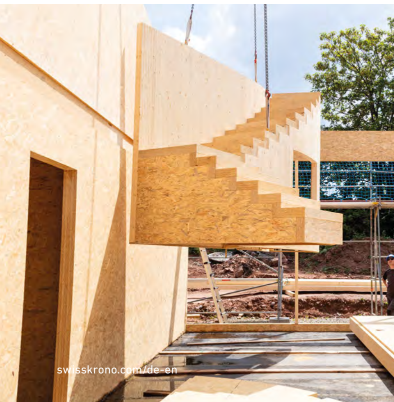
Construction of the RhönKinder-Haus childcare centre in Poppenhausen, Germany
